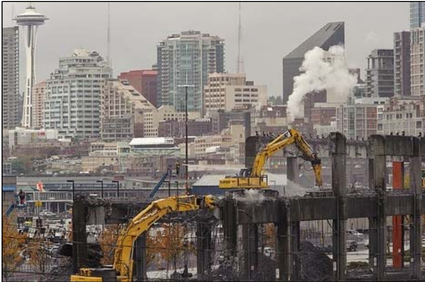
Alaskan Way Viaduct demolition
