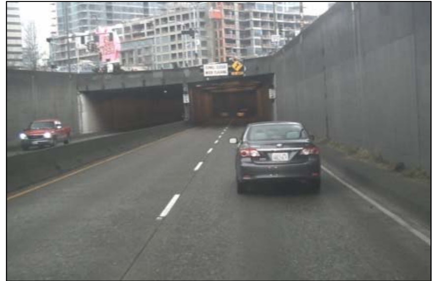
Battery Street Tunnel decommissioning
