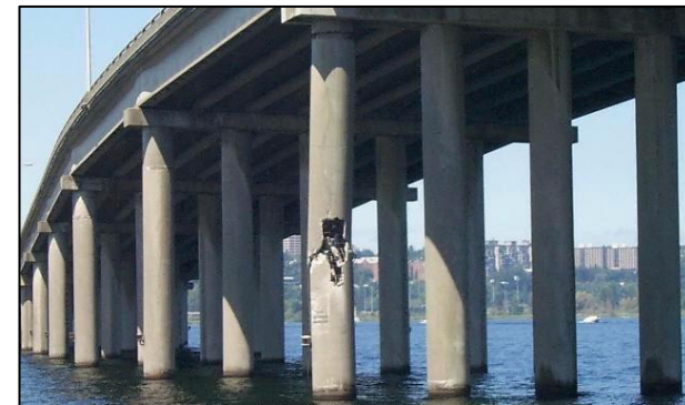
Photo of old, hollow concrete columns for original SR 520 bridge structure.
