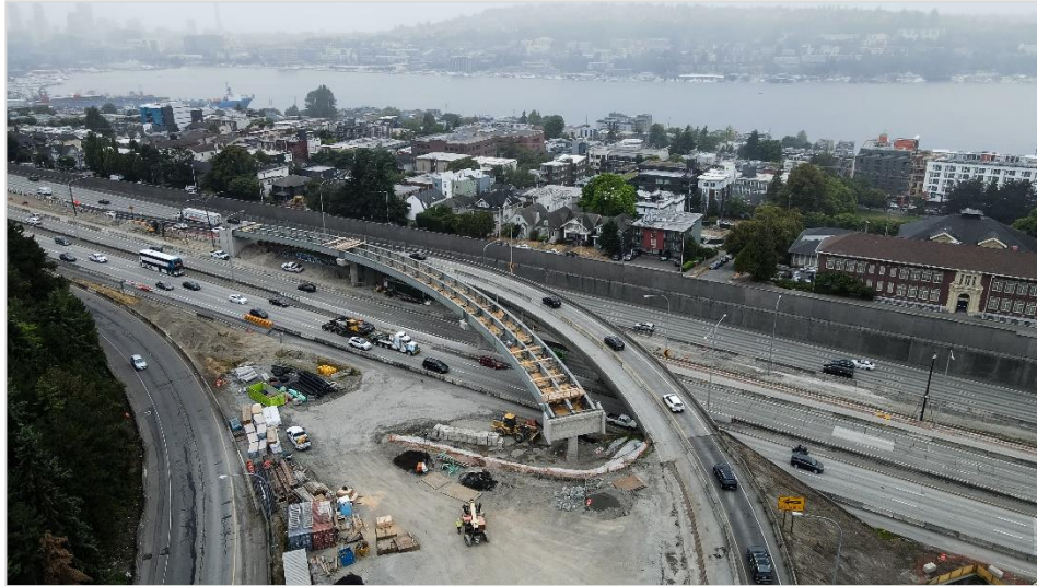
Aerial photos taken in early August showing flyover ramp construction
