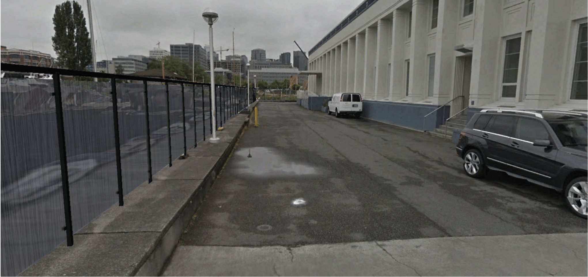
5B - FRITTED SCREENING ALONG THE EAST BULKHEAD
