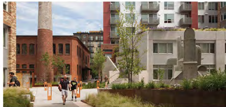
Maintained Scale and Texture With the introduction of 7-12 story office and residential re-development, texture and scale is focused to the lower register, allowing the towers to rise above.
