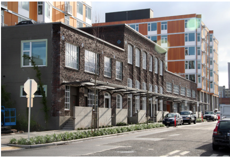
Alley 24 successfully incorporates a Landmark into a new mixed-use project.
