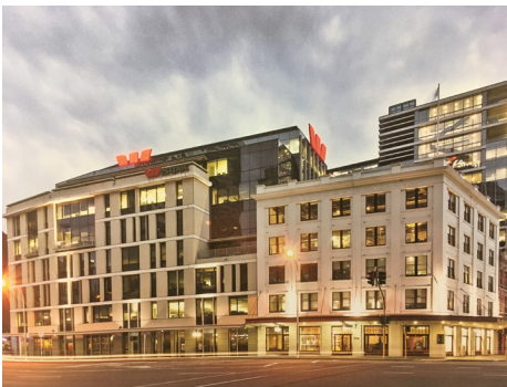
New (left) compatible with restored (right). Taller Portions stepped well back. The Britomart, Auckland, NZ.
