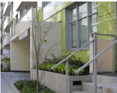
Conceal all underground parking from street views. Planting, artwork, or other uses can effectively screen parking.
